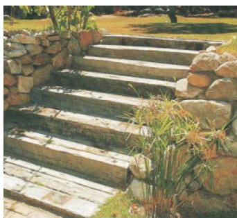
USE OF TIMBER STEPS AND INNOVATIVE TIMBER RETAINING STRUCTURES.
